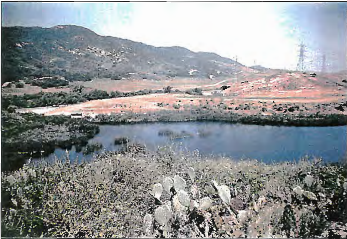
Laguna Lake No. 3 - view from top of buried water tank
