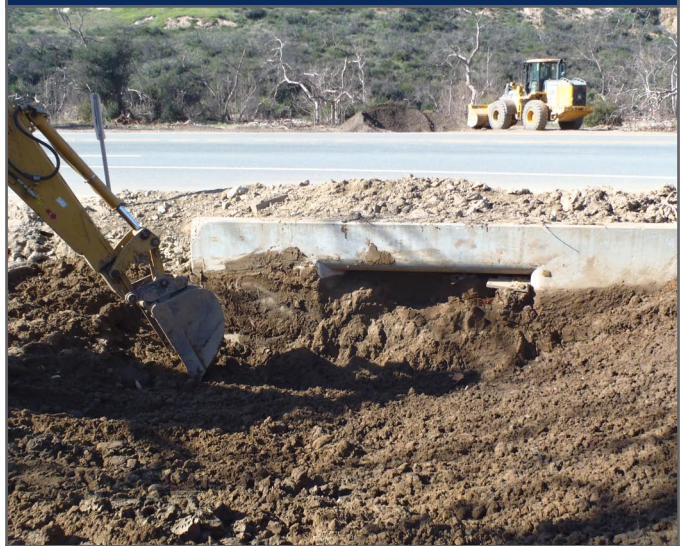
After the rains, Public Works crews dig out a culvert, opening up a vital drainage area.
