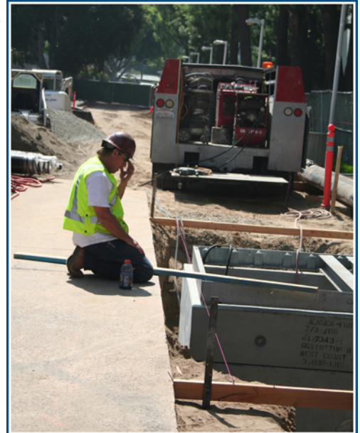
A worker inspects a mechanical vault for steam lines.
