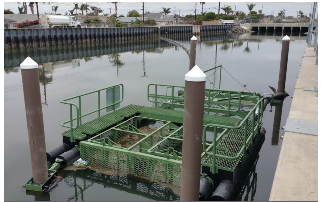
Talbert Channel Bandalong Litter Trap and Boom
