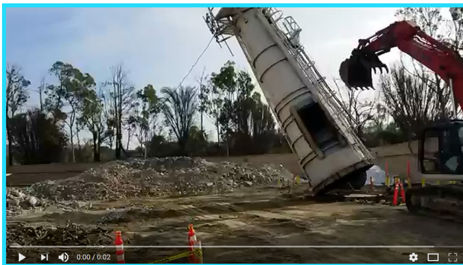
An exhaust stack at the Coyote Canyon Landfill Gas to Energy facility, which was demolished in an effort to remove the facility and make way for a greener future. Photo Credit: OC Waste & Recycling
